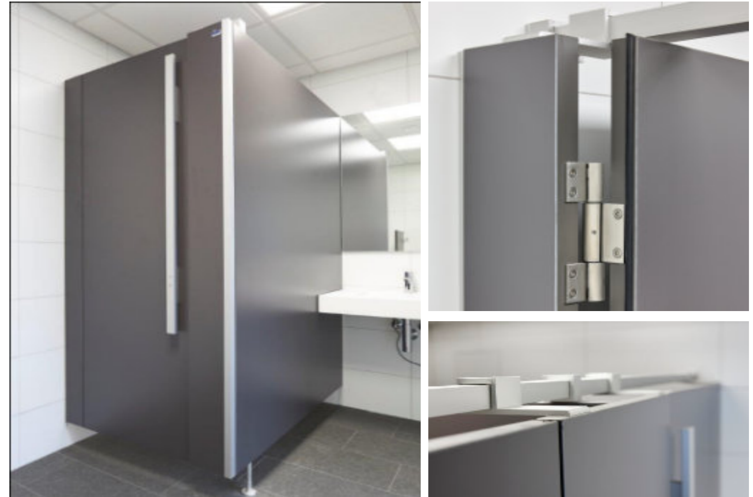
Floating configuration with recessed pedestals and recessed headrail , with wall connection via shadow gap
